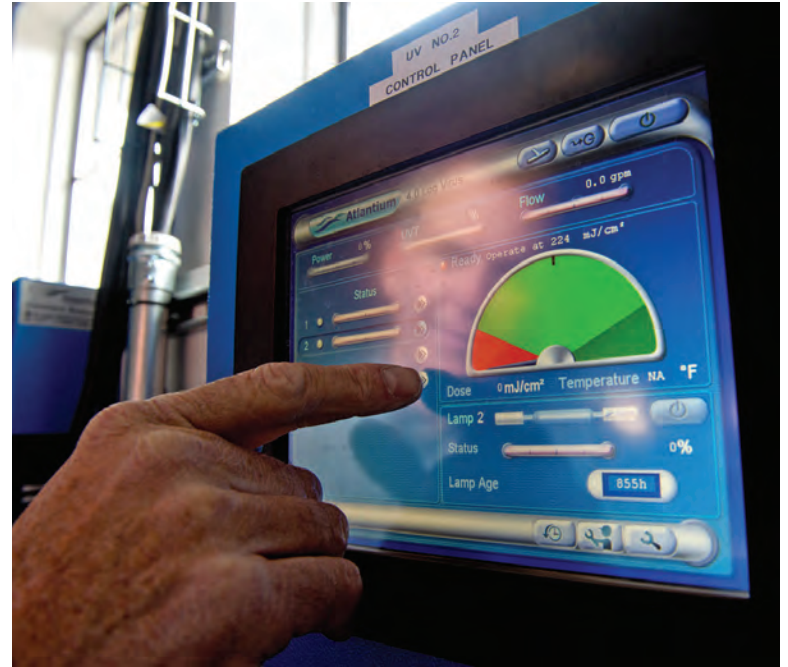
ABOVE/BELOW: Jim Muscat looks after the UV disinfection system (Atlantium Technologies), first of its kind in the state, inside the Spotted Elk Well House.
