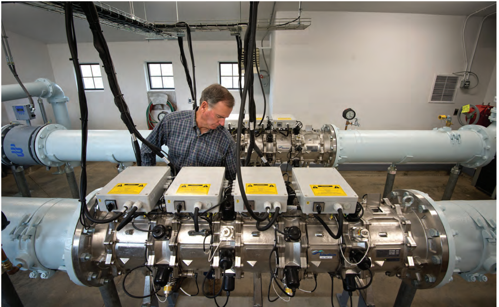
ABOVE/BELOW: Jim Muscat looks after the UV disinfection system (Atlantium Technologies), first of its kind in the state, inside the Spotted Elk Well House.
