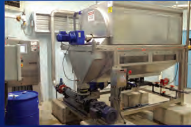
Rotary Drum Thickener
