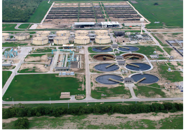
Aerial view of the Dos Rios Water Recycling Center.
