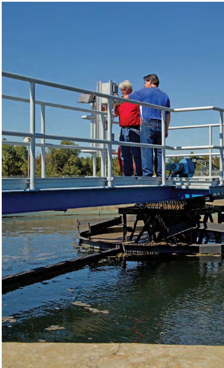
Anthony King (left) and Dean Durham check the status of a clarifier.
