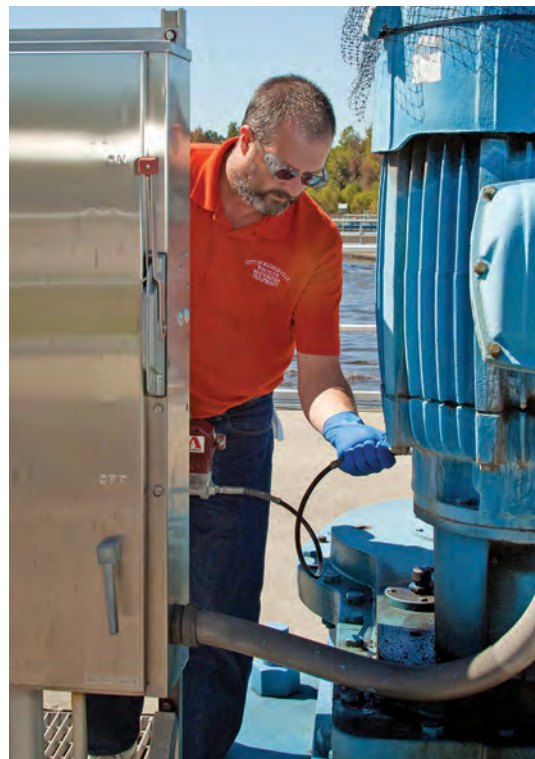
Tim Robards performs a maintenance check on one of the treatment plant’s pumps.
