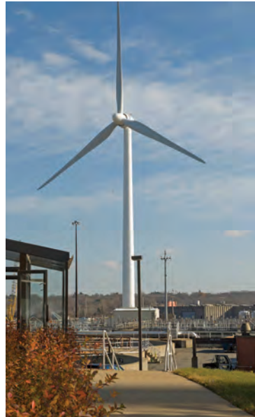
Being near an airport glide path held up the wind project for about 18 months. The Federal Aviation Administration finally allowed 365-foot towers after first ruling they could be no more than 265 feet high. Lower towers would have doomed the project; wind speeds at 265 feet would have been inadequate.
