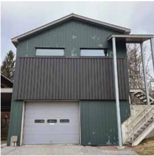
Solar walls like this one help heat buildings at the Essex Junction plant.
