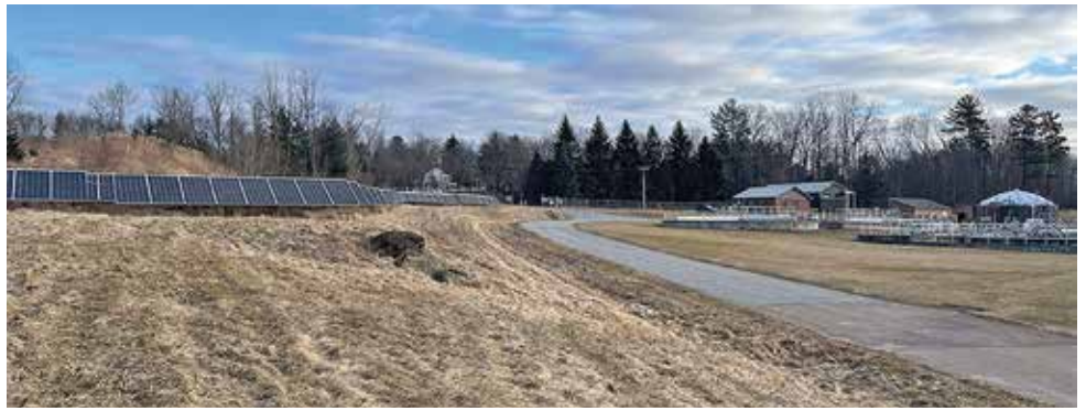
The Essex Junction Wastewater Treatment Facility has a 150 kW array of solar panels.
