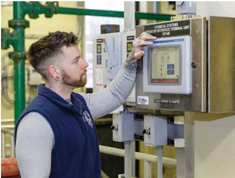
David Milano, assistant superintendent, adjusts the polymer dosing to the belt filter presses.
