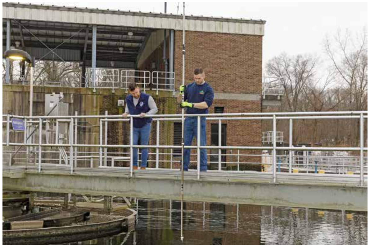
Milano, shown checking final clarifier sludge blankets with Matthew Hannon, enjoys being in control of a process that helps protect the environment.
