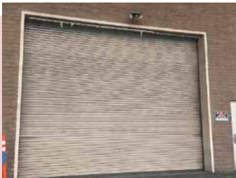
ABOVE: This roll-up door is protected by a security notification horn. CENTER: A pan-tilt-zoom camera is a common security device for facility fence lines.
