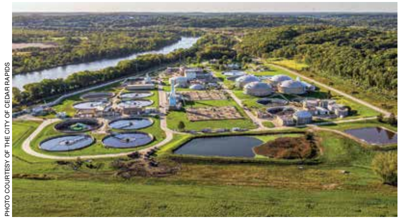
An aerial view of the Cedar Rapids Water Pollution Control Facility.
