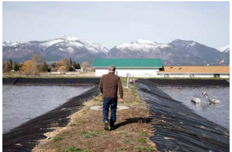
Mosbrucker holds wastewater treatment, water treatment and water well licenses and has worked steadily to improve the Corvallis treatment process.
