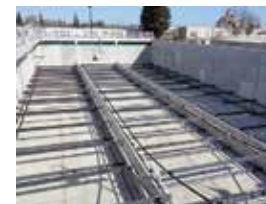
Envirex Chain and Scraper Sludge Collector systems from Evoqua Water Technologies (now part of Xylem)
