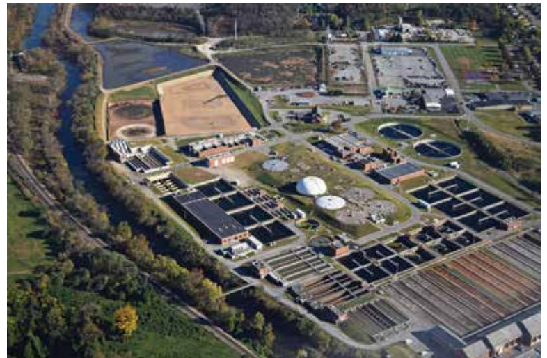
The Roanoke Regional Water Pollution Control Plant treats an average of 37 mgd.
