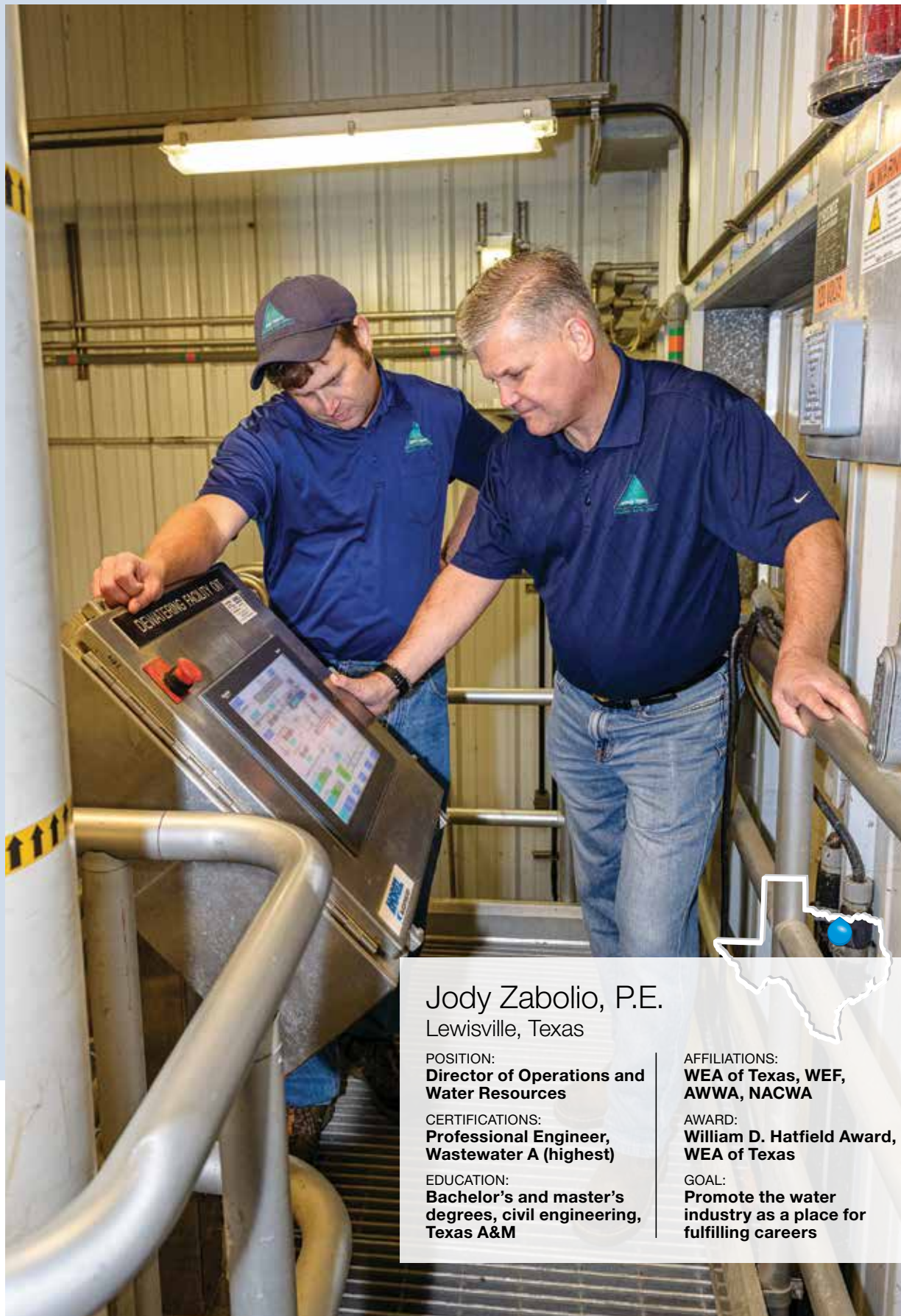
Zabolio, front, and Mark Wootton, senior wastewater operator, review the polymer and solids flow and the torque percentage within the centrifuge in the dewatering building.
