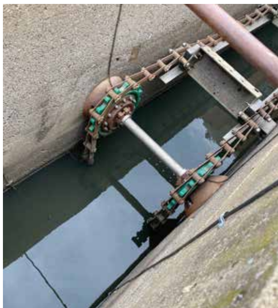
Old-style bearings that had been installed in the grit channel were removed and replaced.
