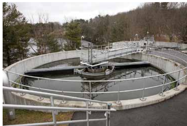
The Newmarket Wastewater Treatment Plant (0.85 mgd design, 0.5 mgd average) uses the 4-stage Bardenpho process.
