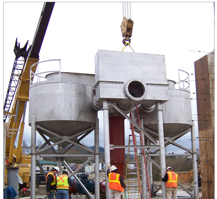
Chehalis Grit King® System During Installation
